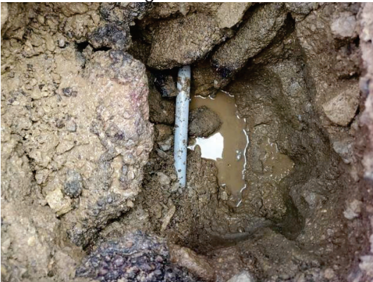
Downhole Looking North
