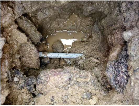
Downhole Looking East
