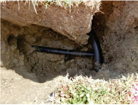
Downhole Looking East
