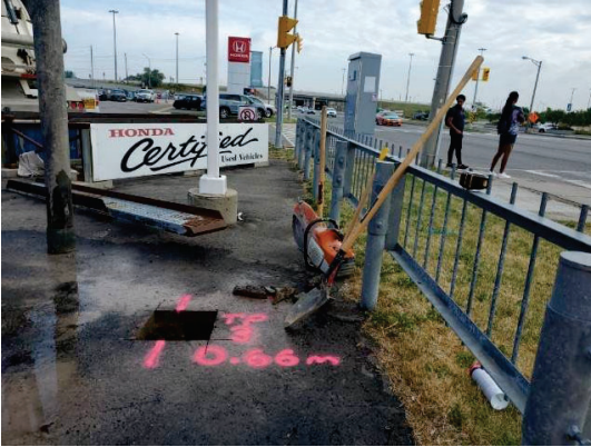
Overview of TP Location
