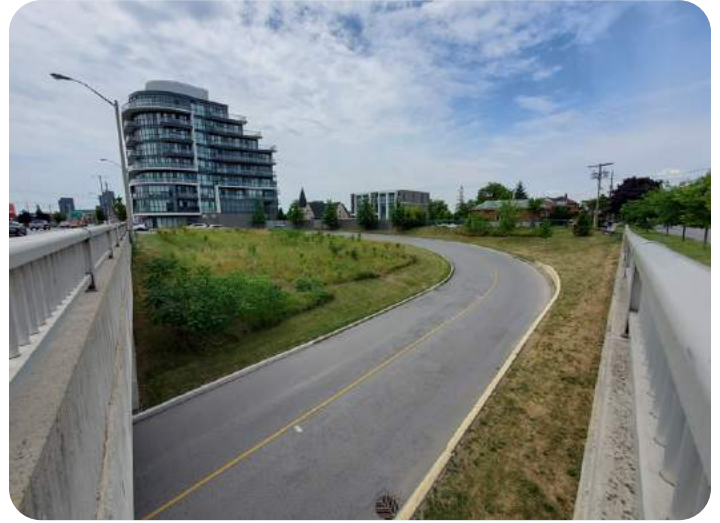
Clover Leaf interchange accessing Yorkdale Shopping Mall
