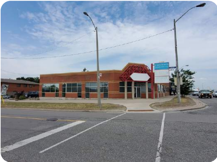
3338 Dufferin Street looking north
