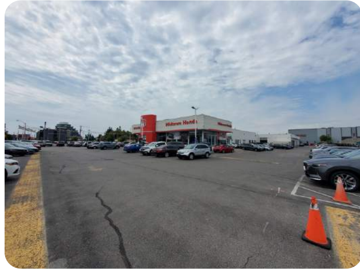
Subject Site looking southwest
