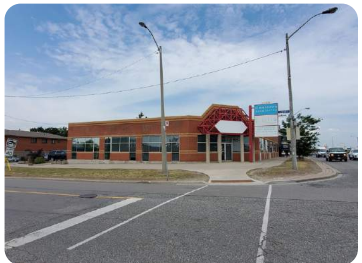
3338 Dufferin Street looking north
