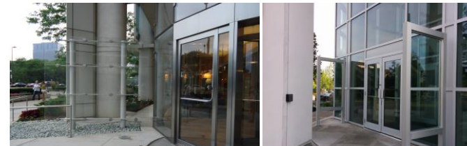
Examples of wind screens near entrances
