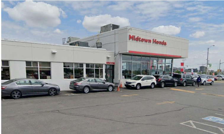
Figure 2a: Looking north at the site
