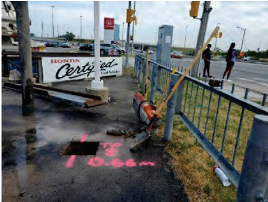
Overview of TP Location
