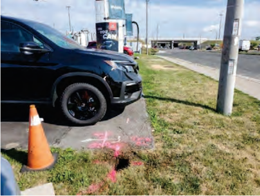
Overview of TP Location
