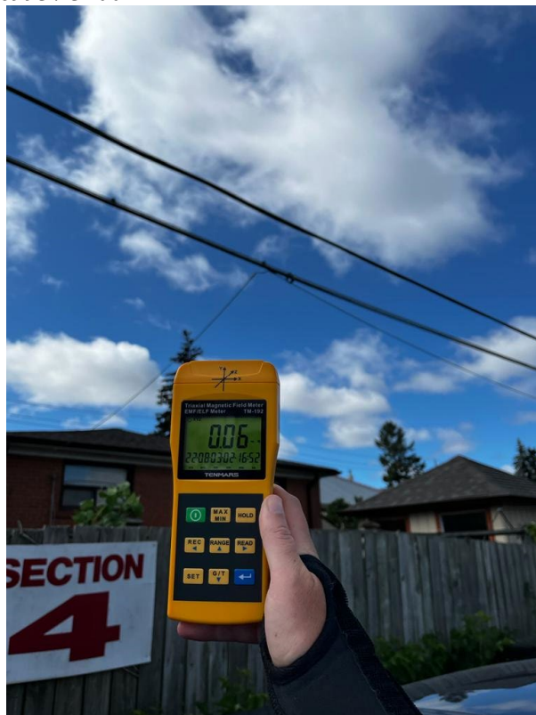
PHOTO #5: Telecom lines running along the South side of the property. Not a source of A.C. magnetic field.
