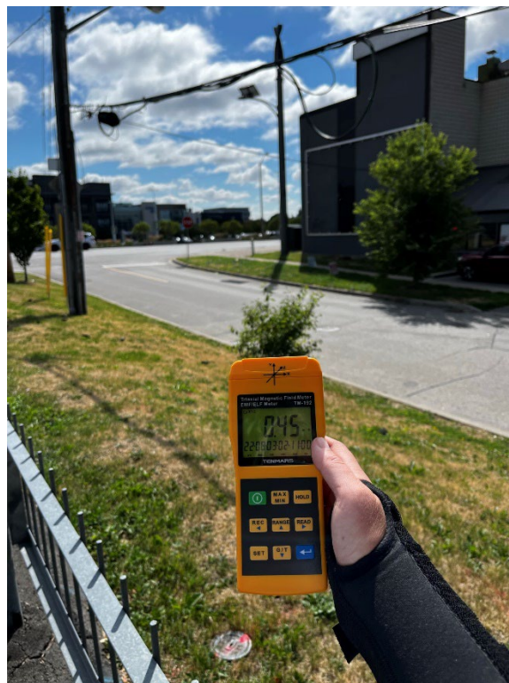
PHOTO #6: City of Toronto distribution lines running along Jane Osler Blvd.
