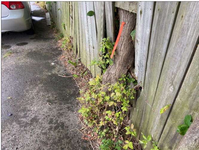
Photograph 4. Example of shared ownership trees (Manitoba Maples) with embedded fence and asphalt over roots (TPZ) (July 5, 2022).
