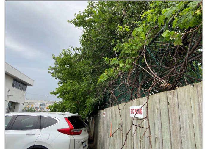
Photograph 3. Representative of tree locations and driplines along the subject property boundary (July 5, 2022).
